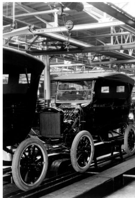
Model T automobiles roll off the assembly line at the Ford Motor Company in Detroit, ca. 1920s.
